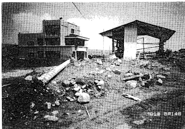
Photo 1: Flood damage at Mujiliao Village
