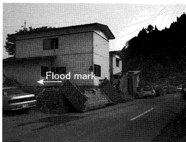
Photo 4 Inundated house in Higashiyama Town. Inundation by over flow in spite of being built on filled ground (about 1m). The wall was destroyed the river water. Photos 4, 5, and 6 were taken on July 13 by the author.
