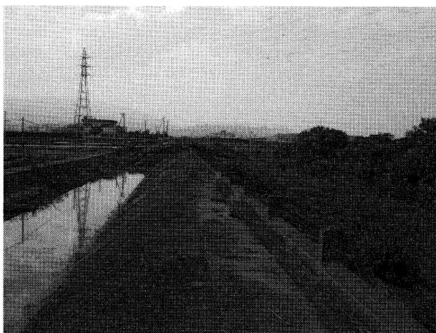
Photo 2 Close-up of the fuse plug levee (Otani River Arai zeki).
